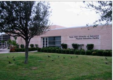
Campus buildings are currently identified with three types of signs: (I) a 5-foot by 2-foot facade-mounted metal panel, painted maroon with reflective white vinyl alpha-numeric designations in a I-foot capheight; (2) individual letter forms, painted black, mounted to the face of the building, and (3) white vinyl mounted to glazing adjacent to building entry doors.
